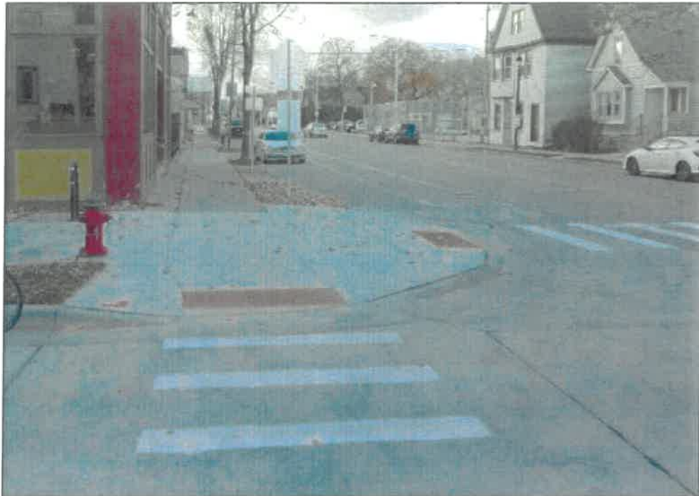
Figure 5-5 Traffic Calming Bump Outs
