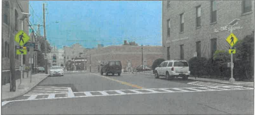
Figure 5-7: Typical RRFB Installation at an Intersection
