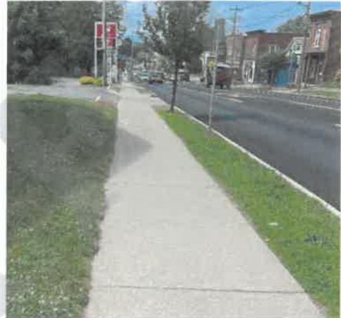
Typical Roadside Condition Near 3 rd St.
