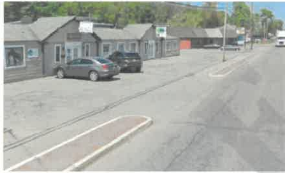
Figure 2. Segment between Feeder Dam Road and Beach Road
