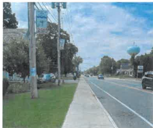
Existing Sidewalk Adjacent to Stewarts
