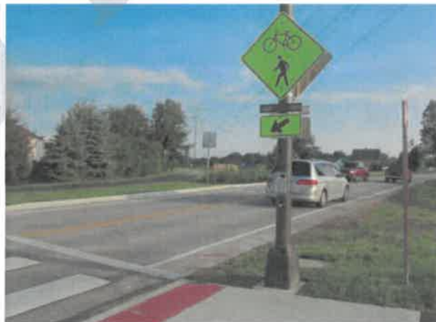
Figure 5. RRFBs Used at a Crossing. Source: FHWA
