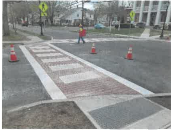
Figure 4. Imprinted Thermoplastic Crosswalks. Source: Harbour Roads and Ennis-Flint
