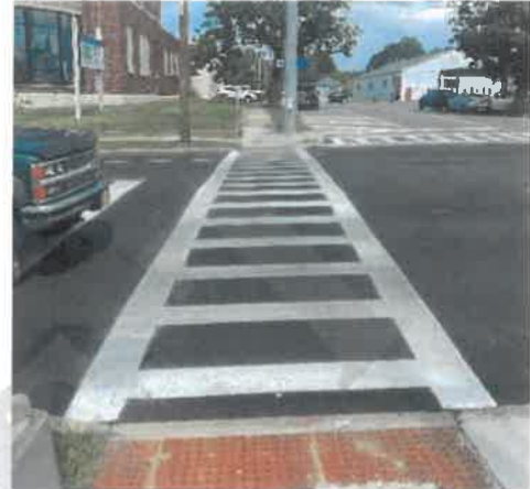
Pedestrian Crossing at 3 rd St.
